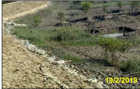
Sandbags protected by bamboo piles Chandipur
