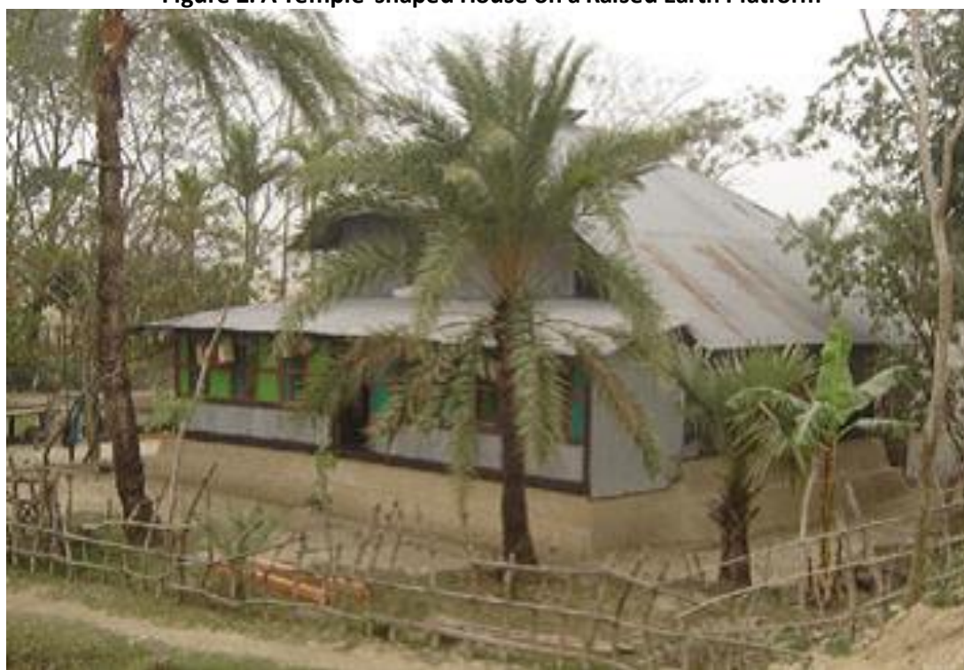
Figure 3: A House Designed to Face Less Wind Forces During Cyclones (Gentle Sloping of the Roof of the House)
